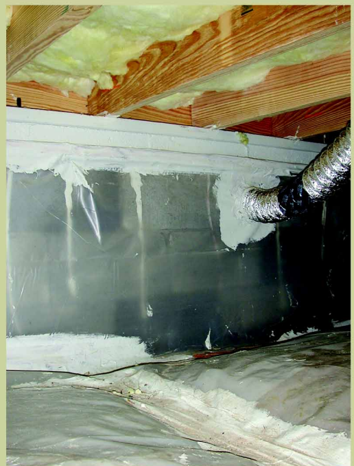
Figure 1 (top). This wall-insulated closed crawl space uses 2-inch thick, foil-faced polyisocyanurate insulation. The foam plugs in the band could be replaced by sections of R-19 batt insulation. A termite inspection gap is visible at the top of the wall insulation.
