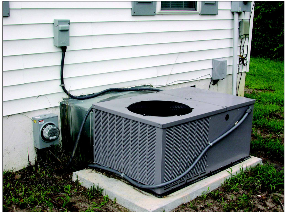
Figure 6. The sub-meter that measures electricity used by this heat pump is visible to the left of the duct cowling.
