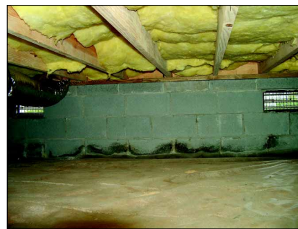
Figure 5. The wall-vented control houses in this study are much better than the typical crawl space we encounter in the field. They have well-installed insulation and 100 percent ground vapor retarder coverage of the soil, and no problems with intrusion of liquid water from outside.
