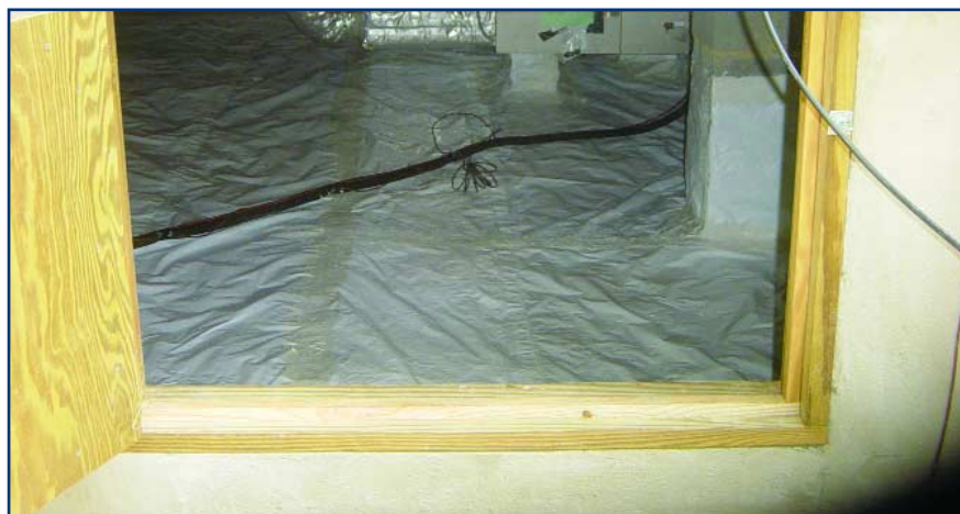
The entrance to this closed crawl space is elevated well above exterior grade, reducing the likelihood of water entry in heavy rains or minor flooding. Photo credit: Indoor Environmental Systems.
